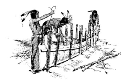
When all this has been done, every seam, or hole made by the needle, is covered plentifully with pitch from the pine tree, which is not unlike soft tar, and when it has been thoroughly dried, you have a boat that will support from two to six persons, while yet so light that one may easily carry it on his shoulder.
